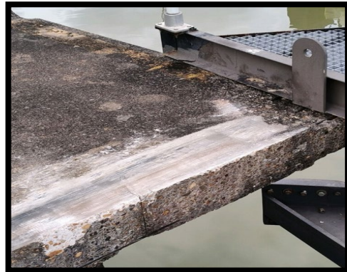
Gate Resting on Concrete Recess as Result of Hinge Assembly Failure
